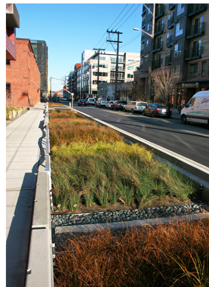
Seattle is using LCLIP revenues to improve mobility, transit, and streetscaping in its urban core with projects similar to this bioswale.
